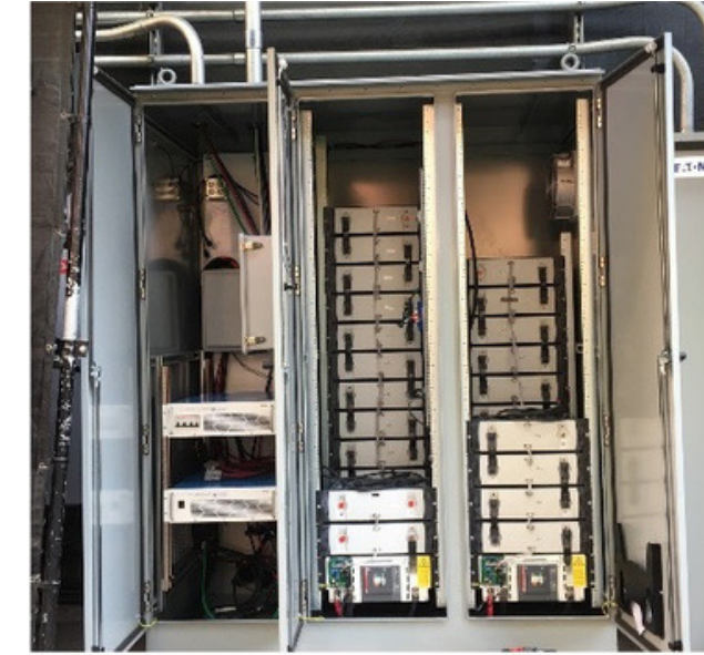
56 kWh Saft BESS in PS 9
