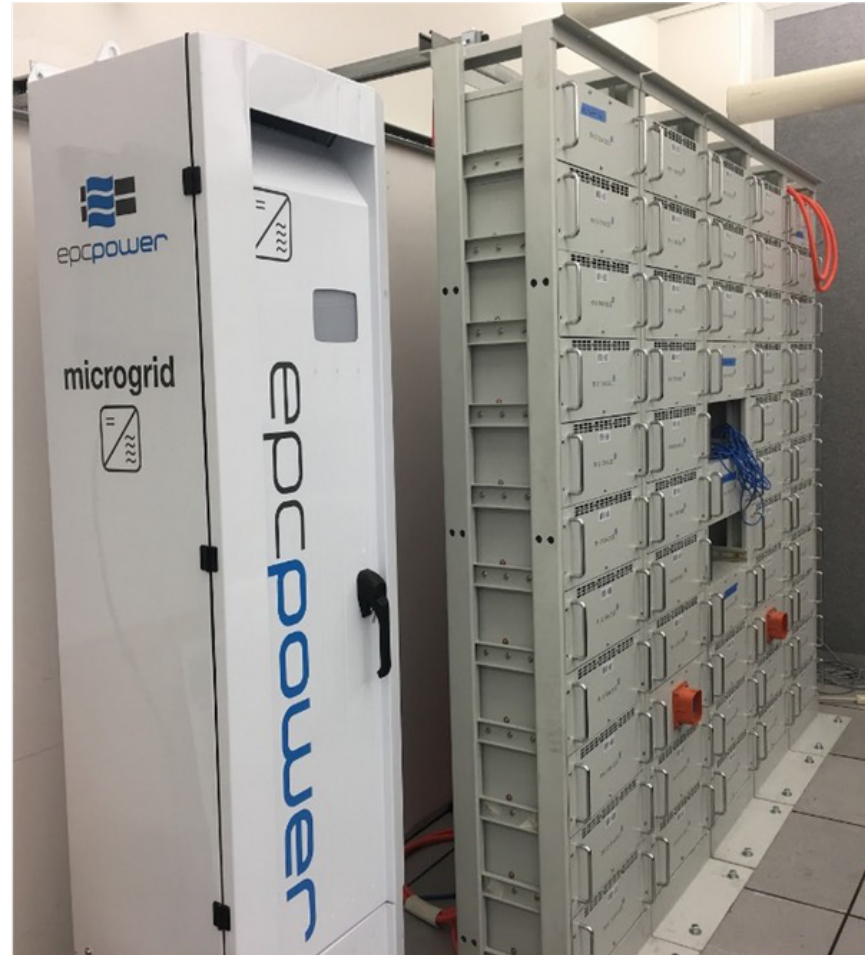
Microvast Li-ion Battery with EPC Power Inverter
