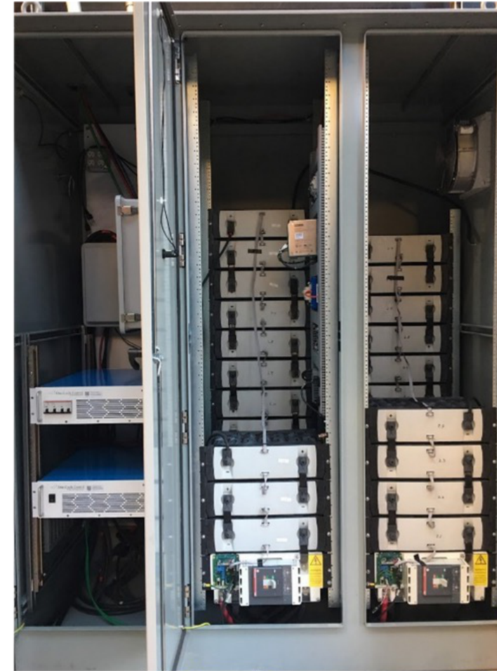
Saft Li-ion Battery with OCC Inverters
