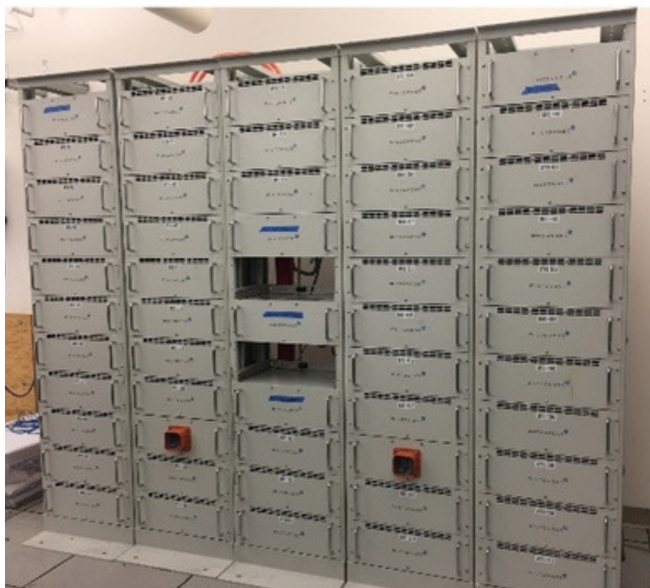
50 kWh Microvast Li-ion Battery with EPC Power Inverter
